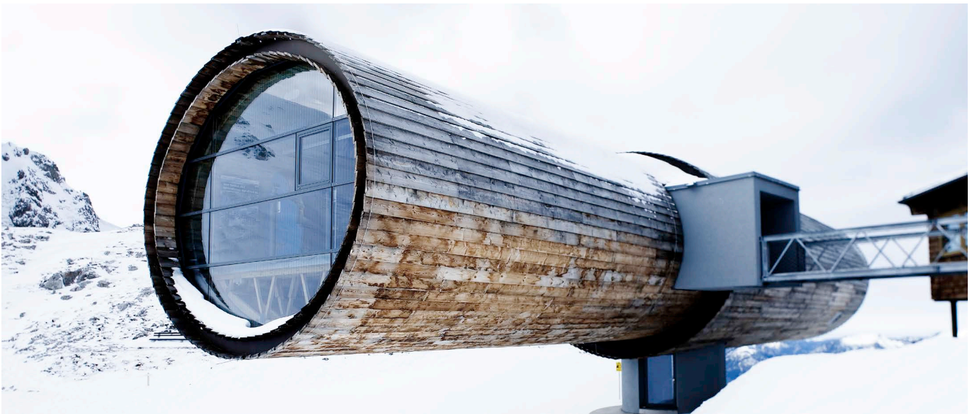
Mountain station Karwendel, Mittenwald Germany
