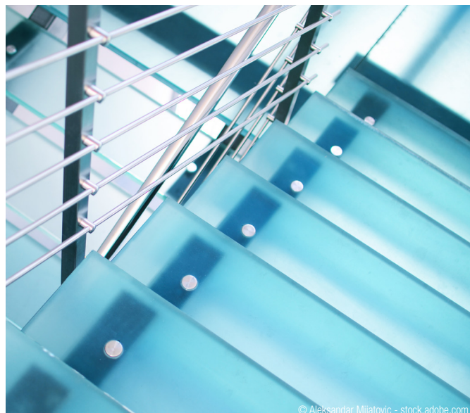
Stair treads consisting of laminated safety glass.
