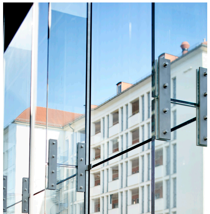
Thermally toughened safety glass by arcon® at Busmannkapelle Dresden, Germany.
