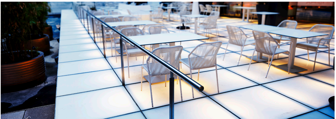
Walk-on terrace made of laminated safety glass in the Amici restaurant, Stuttgart.
