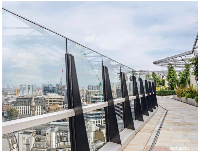
Fall-proof glass railing on a house roof.
