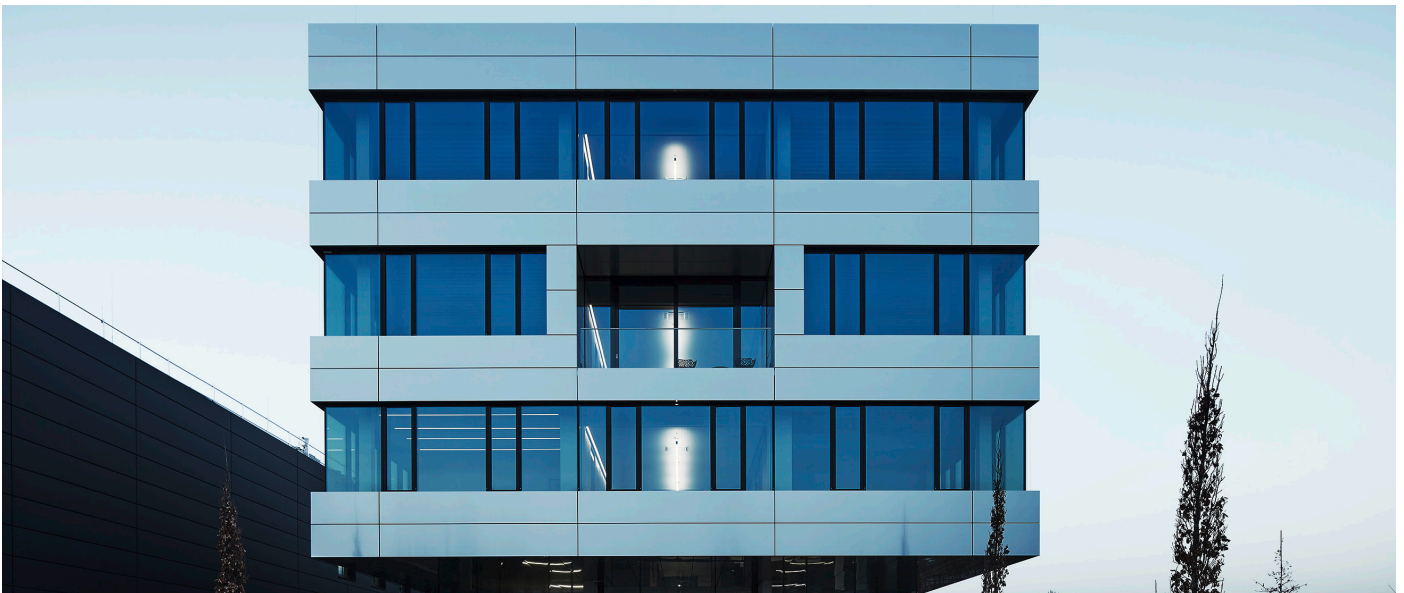
sunbelt® A60 in the corporate office building of Fischer Kälte-Klima near Stuttgart, Germany.
